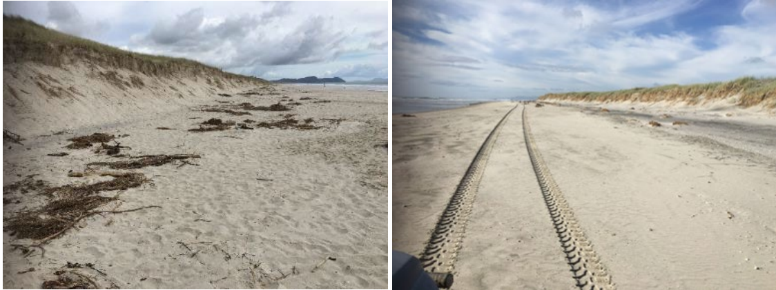
Figure 4-6. Open coast beach front about 1km south of the tip of the spit where the dunes are very eroded. Images taken 28 March 2023 following Cyclone Gabrielle.
