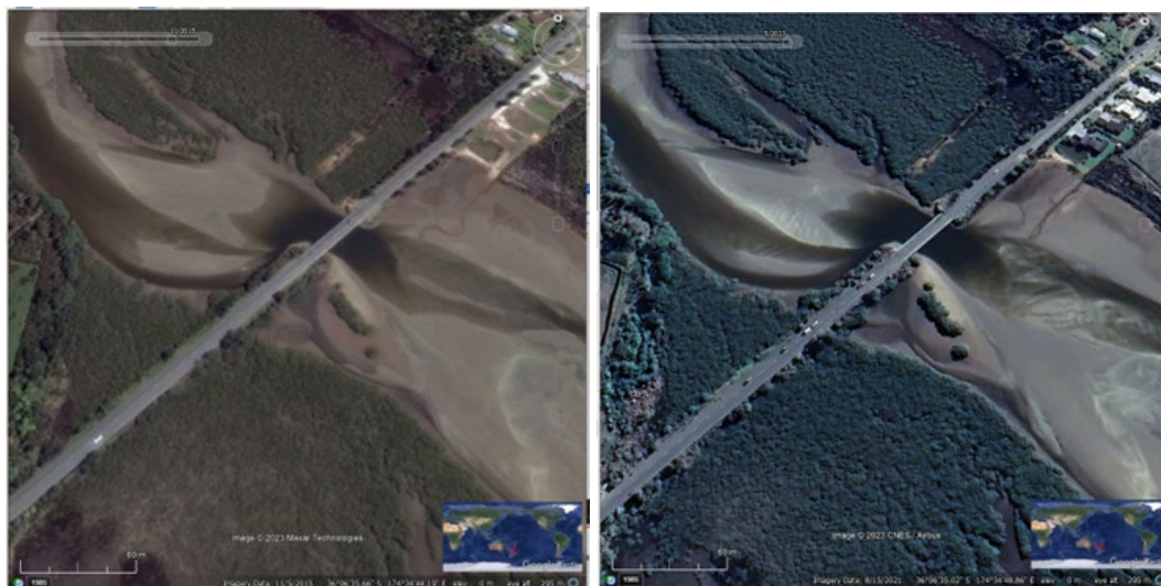
Figure 4-4 Changes in channel morphology in the vicinity of the Molesworth Drive northern causeways. (Source: Images from Google 2015 and 2023).
